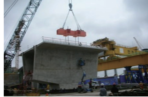
> Lifting Device 설치
